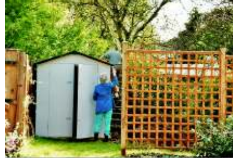
Installing the shed
