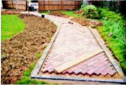
Laying the path
